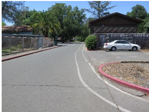
Figure 18 “Secondary Zone” painted sidewalk
