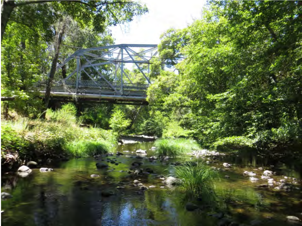
Looking downstream at South Sonoma Creek crossing
