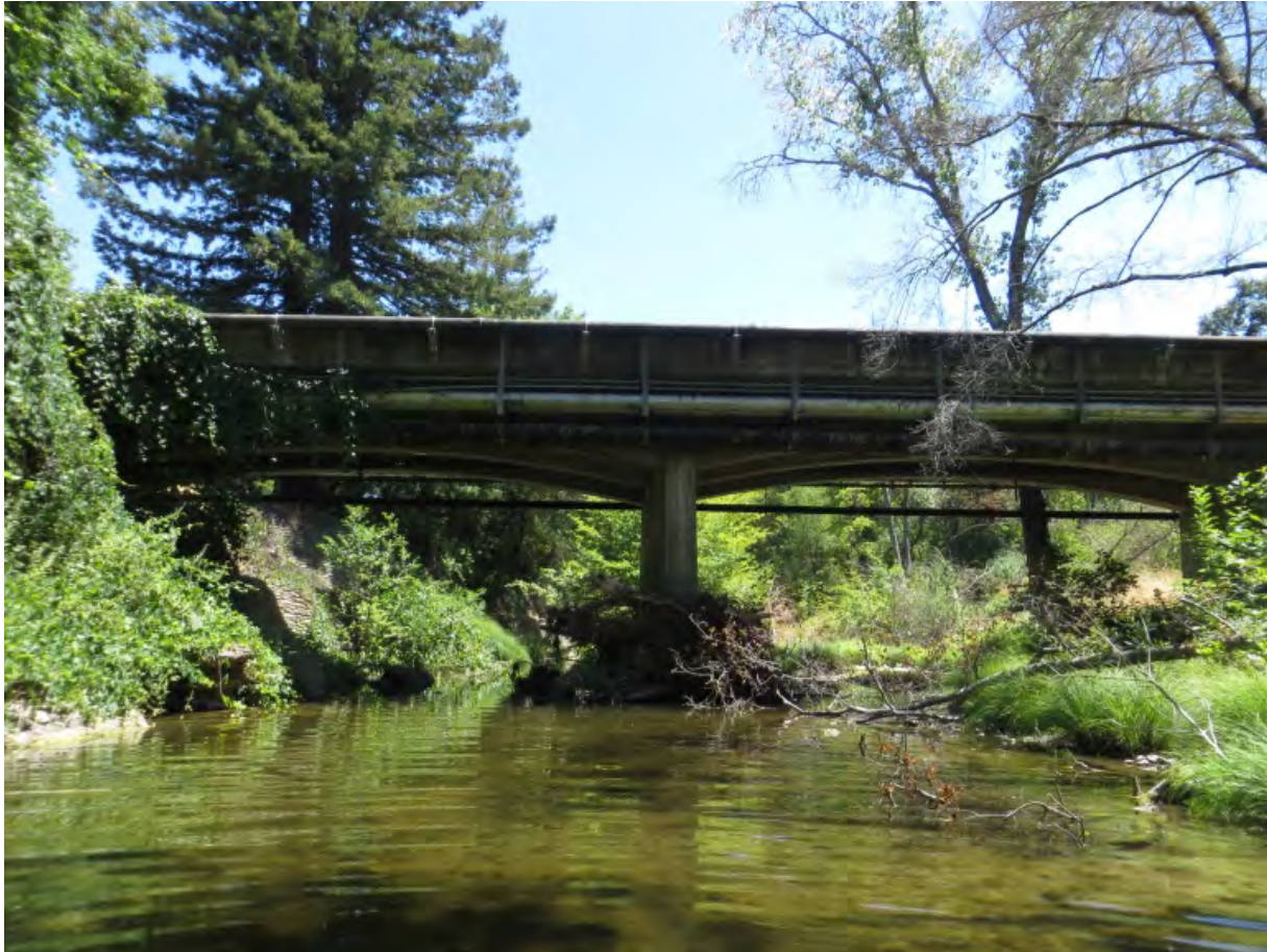
Looking downstream at Sonoma Creek crossing at Harney Drive
