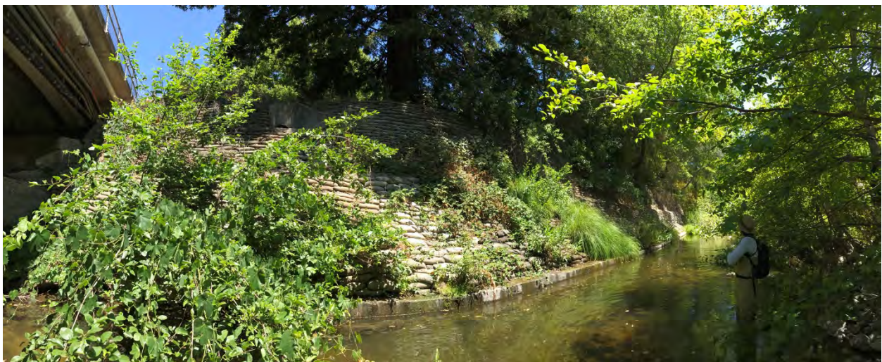
Concrete bag retaining wall downstream of the Harney Drive crossing.
