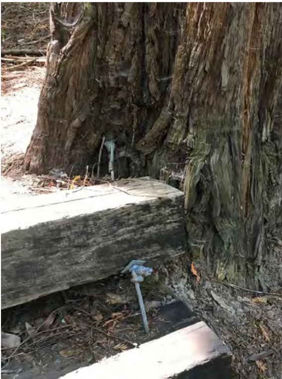
Attachment of stairs to redwood.
