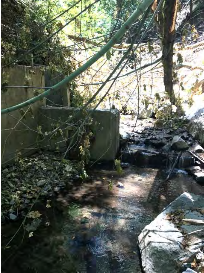
Looking upstream at diversion.
