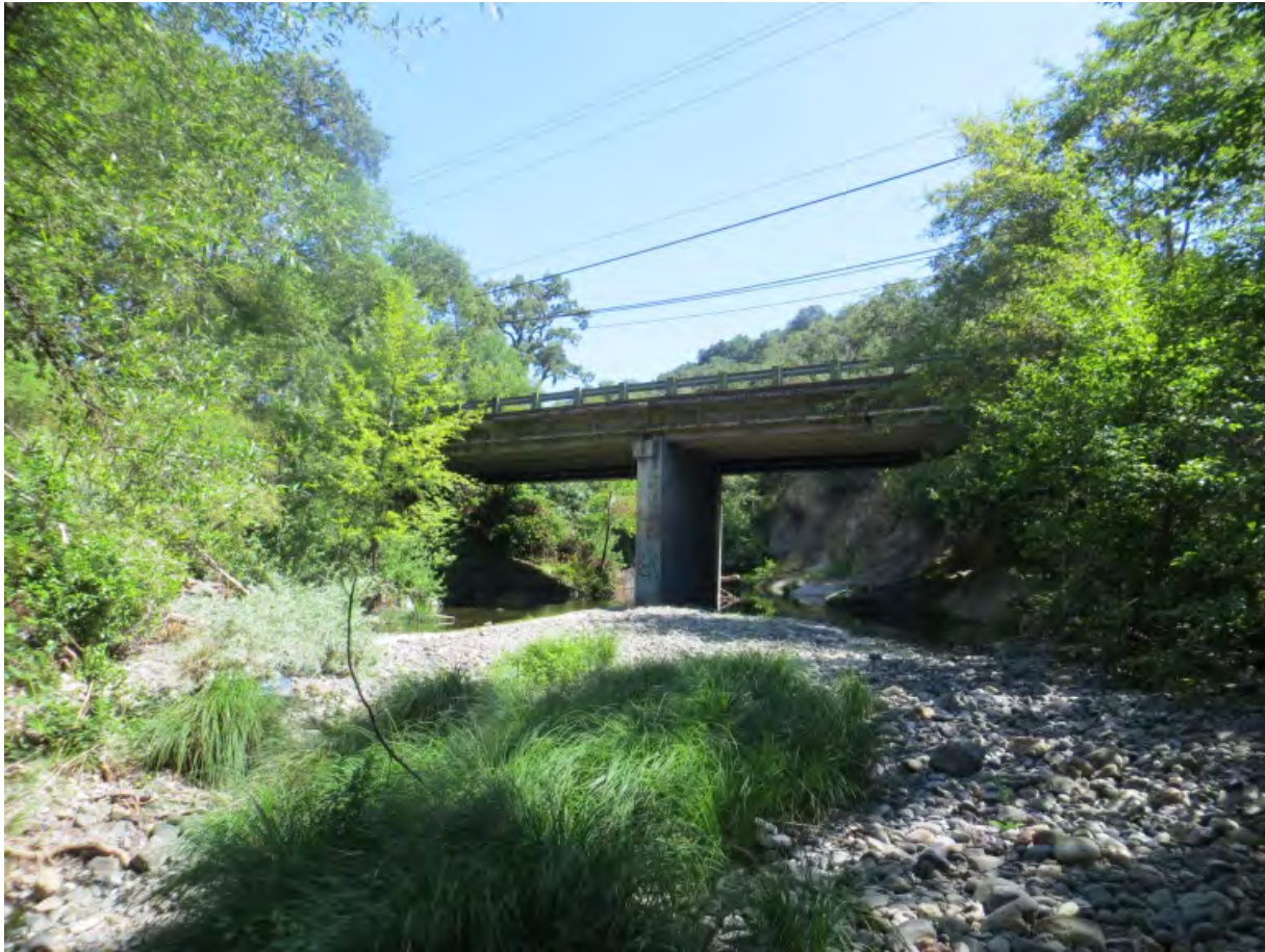
Looking upstream at North Sonoma Creek crossing
