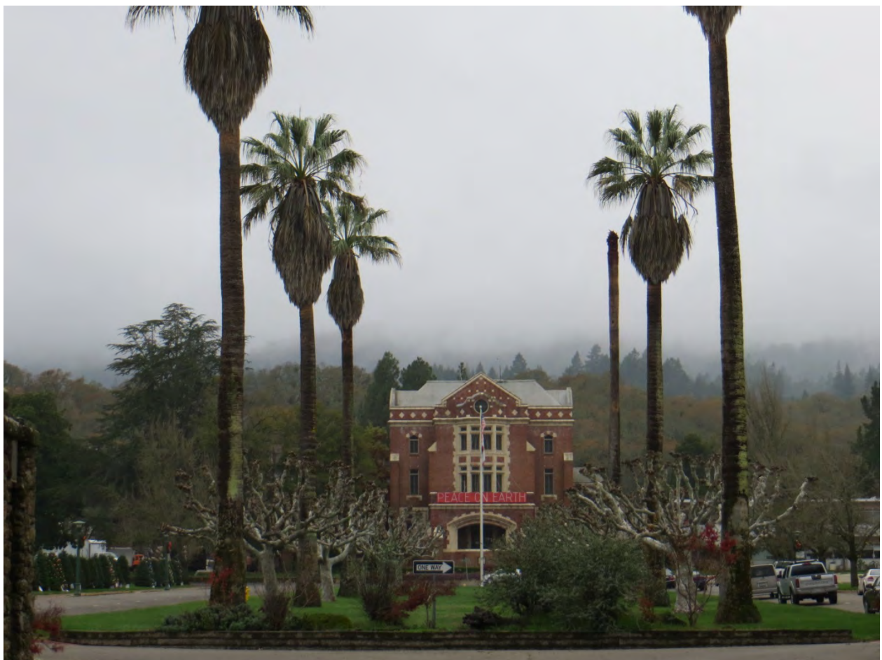
View into the property from Harney Drive entrance to the southwest.
