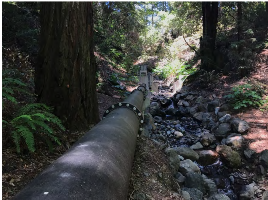
Asbury Creek diversion structure and pipeline to Fern Lake.
