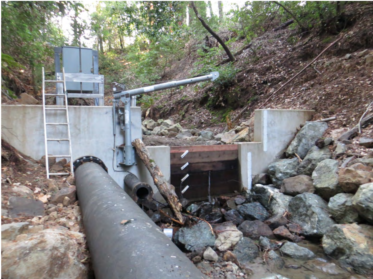
Diversion and dam.
