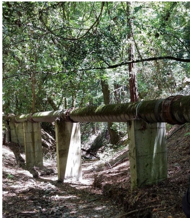
Photo 3: Hill Creek Pipeline.
