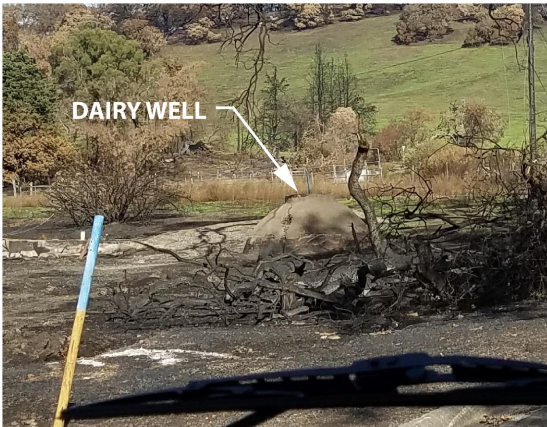
Photo 5: Dairy Well (after the fire).
