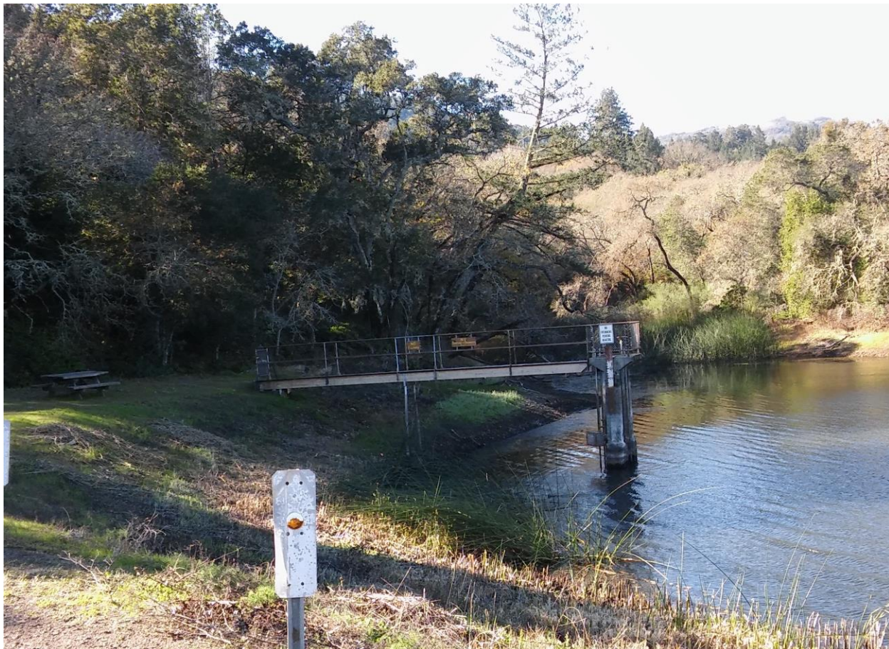
Photo 6: Intake at Fern Lake.
