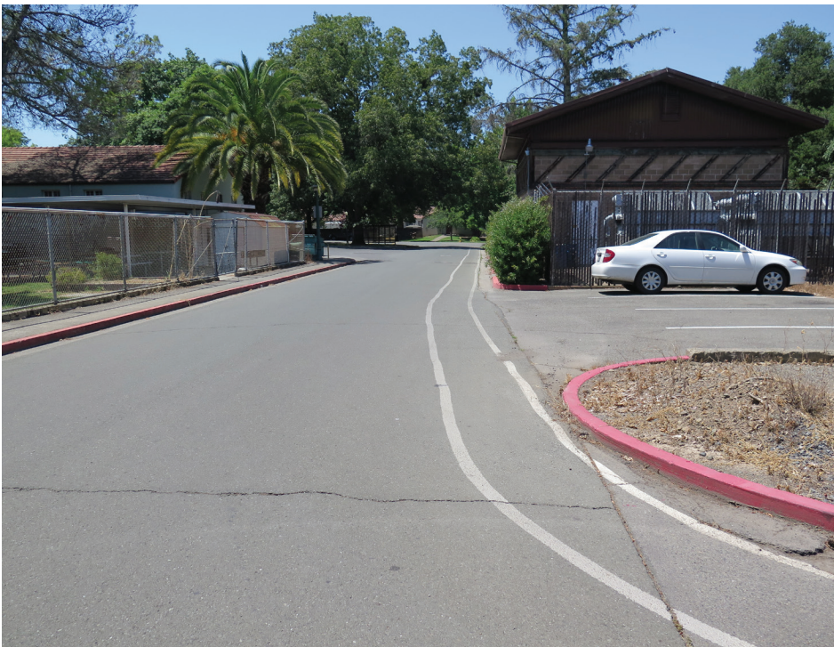
On-street parking along internal streets on the SDC site (top). Painted sidewalk (bottom).
