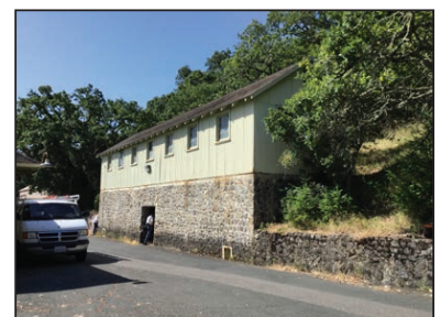
PLUMBERS/MOTORPOOL STORAGE (ca. 1926-1931)
