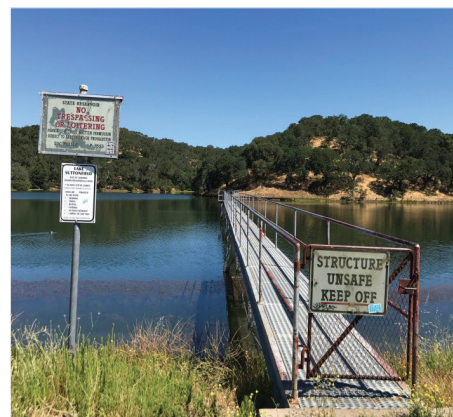
Fern Lake prohibitions (top). Warning signage at Suttonfield Lake (bottom).
