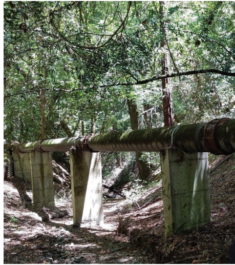
Photos of the Hill Creek diversion weir (left) and the diverted water pipeline over the culvert that carries the streamflow (right).
