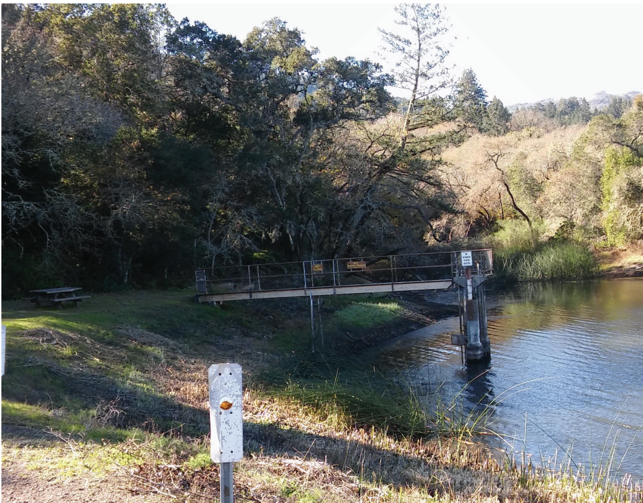
Intake at Fern Lake
