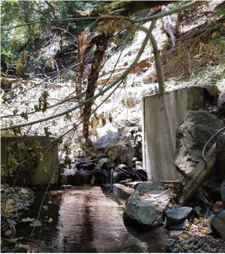
Photos of the Hill Creek diversion weir (left) and the diverted water pipeline over the culvert that carries the streamflow (right).
