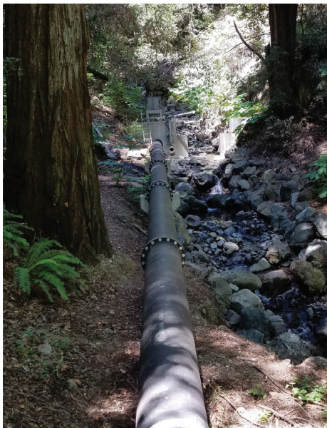
Photo of Asbury Creek diversion (left) and flow monitoring equipment (right: Asbury data recorders). Note the small pipe opening in the weir wall designed to allow 0.9 cfs stream flow to bypass diversion.
