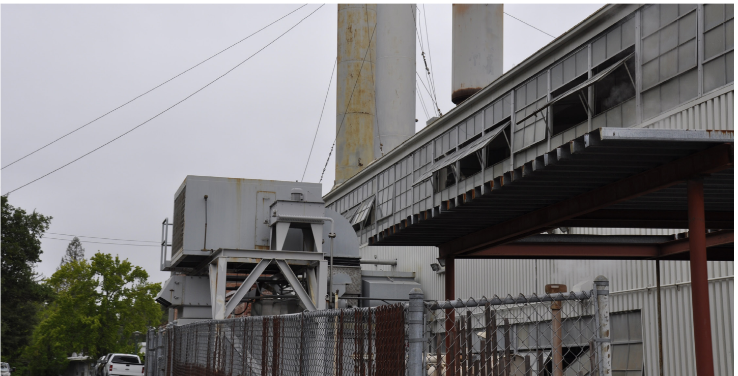
Central Utility Plant
